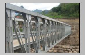
Designed as a permanent structure, the Liberty Series Bridge can also be used as an emergency or temporary bridge. And when the time comes to move it, simply unbolt and move it in desired lengths to other locations. Comprised of 8' wide x 12' high welded panels fitting into top and bottom channel guides, the Liberty Series Bridge is easy to configure, install and maintain with no need for special equipment.
