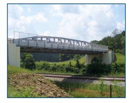
An all bolted, galvanized U.S. Bridge® Cambridge style vehicular truss bridge was used to link the soccer fields. A 5-ft.. exterior sidewalk was installed on one side for pedestrian access. Floor beams were raised into the structure, allowing the required railway clearance while not increasing the need for additional approach road grading.
